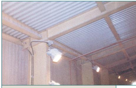
**Figure 7:** Potash plant, raw ore storage interior. A hot and humid potash environment containing potash dust. Note potash build-up on light fixtures. Eleven years exposure in Saskatchewan.
