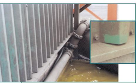
**Figure 1:** Mine water cooling tower. West exposure above the tanks. Insert: A quick cleaning showed that the drip edge was in excellent condition. Eleven years exposure in Northern Ontario.
