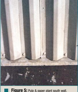
Figure 5: Pulp & paper plant south wall, upper elevation of recovery boiler building. Eleven years exposure in Northern Ontario.
