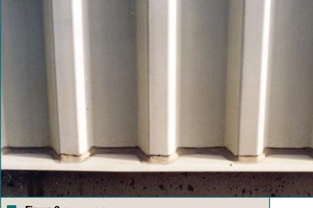
**Figure 9:** Example of effective edge sealing with caulking on an exterior wall.
