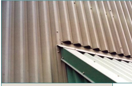
**Figure 2:** Mine smelter building exterior. Base edge and 45° angled cladding exposure. Nineteen years exposure in Northern Ontario.
