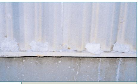
**Figure 4:** Pulp & paper plant, recovery boiler building. Ground level west exposure below exhaust duct showing contaminate build-up and minor edge creep on the cladding. Eleven years exposure in Northern Ontario.
