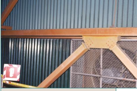
**Figure 3:** Mine refinery building interior. The Barrier Series cladding is above the exhaust fan. Eleven years of exposure in Northern Ontario.
