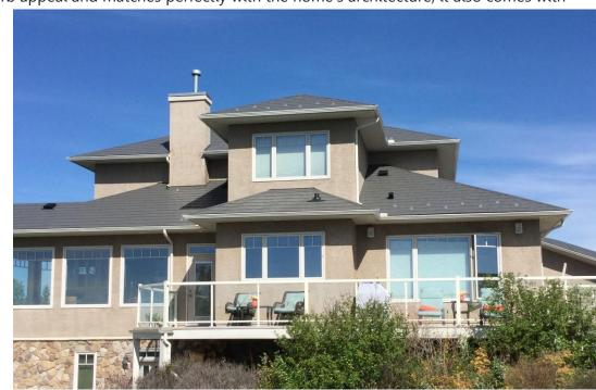
job also was essential to help ensure maximum performance. Installers from GBH Enterprise in Alberta made sure no detail was overlooked, including installing a heavy duty membrane underlayment to the plywood prior to applying the steel roofing which adds an extra layer of protection.
