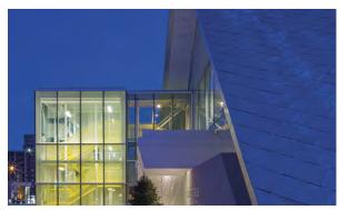
Both the spire and the roof were stripped and re-clad with Galvalume Plus<sup>TM</sup> corrosion resistant steel, arranged "à la Canadienne", in an overlapping 45-degree pattern. The attractive bright appearance and reflectivity of the roof in all weather conditions is one of the new library's most striking features.
